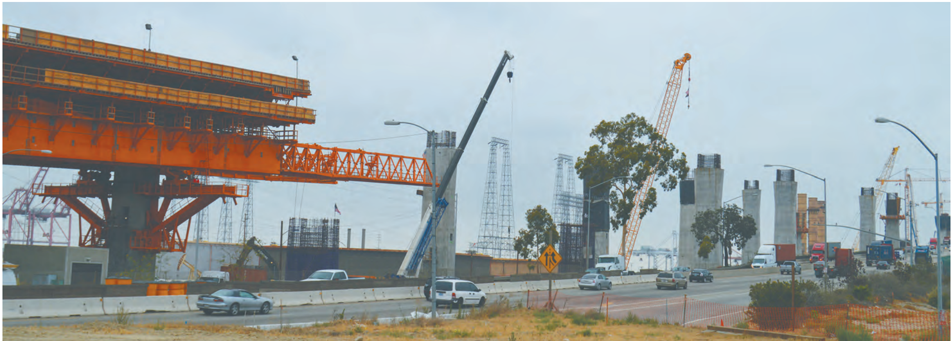
The Port of Long Beach is in the midst of a years-long project to replace the Gerald Desmond Bridge. The new bridge is being built alongside it. Its columns and towers have already surpassed the height of the existing bridge, and a moving scaffolding system has completed three segments of one of the bridge’s approaching ramps. The new structure is being built higher to let larger vessels pass beneath it. (Photograph by the Business Journal’s Larry Duncan)
