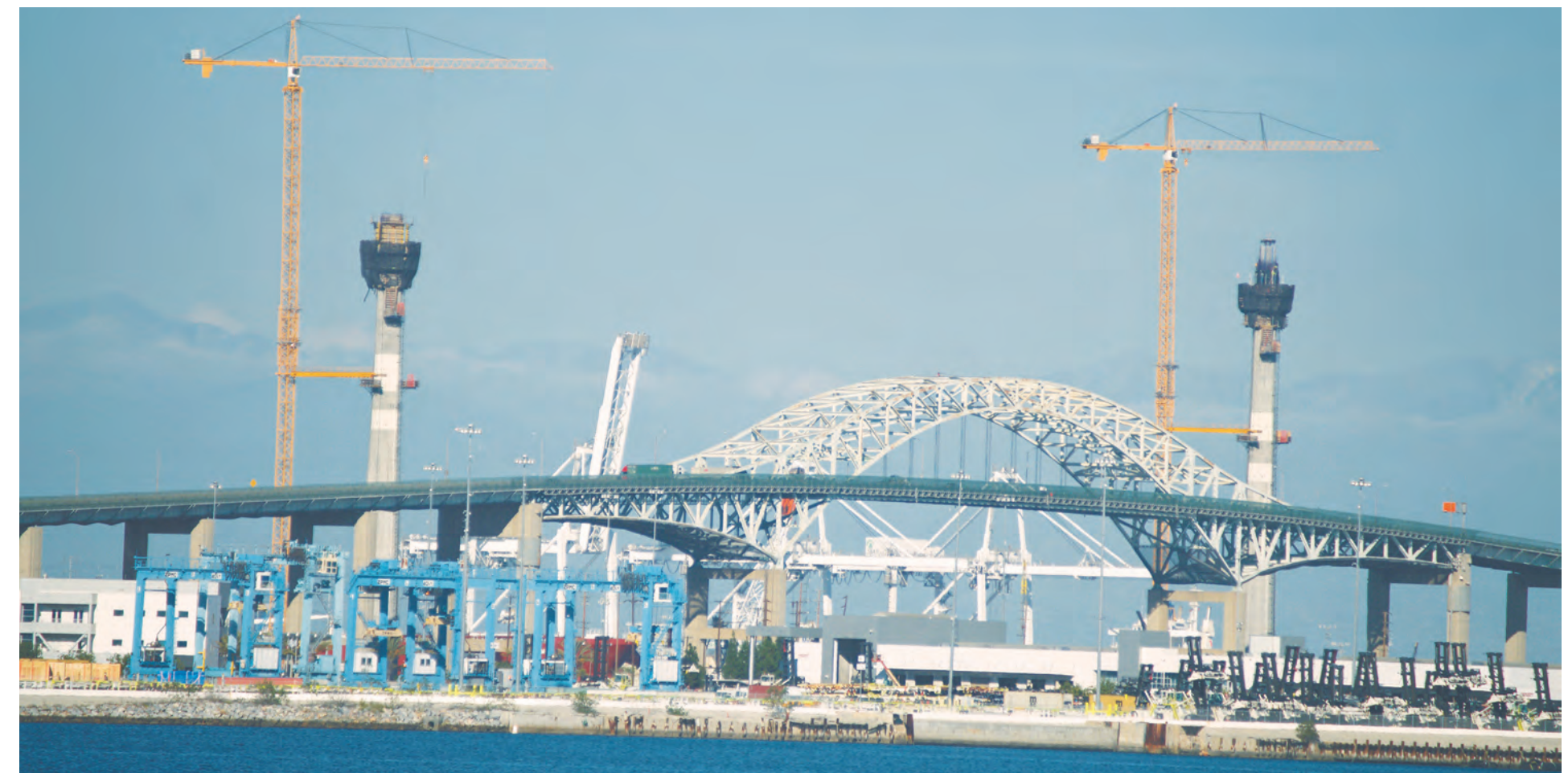
Construction on the replacement for the Gerald Desmond Bridge continues at the Port of Long Beach. When completed, its roadway will be about as high as the top of the arch on the current bridge – about 200 feet. According to port spokesman Lee Peterson, the two towers that will support the cable stayed span of the new bridge will each be 515 feet high. The clearance over the water for the current bridge is 155 feet. For the new bridge it will be about 205 feet, allowing larger vessels to pass beneath it in to the inner harbor. The new bridge will also feature more lanes for traffic. (Photograph by the Business Journal's Larry Duncan)
