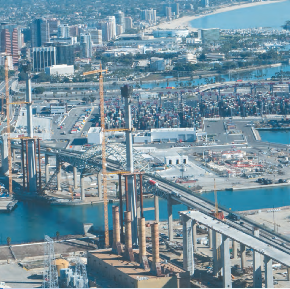
The Gerald Desmond Bridge Replacement Project is one of the Port of Long Beach’s major capital improvement undertakings. At right is the existing bridge. At left, the new bridge’s columns have been built to their full height, making them the tallest structures in Long Beach. The bridge is being built with a higher clearance above the water to allow larger ships into the inner harbor. (Business Journal photograph by Evan Patrick Kelly, December 6, 2017)
