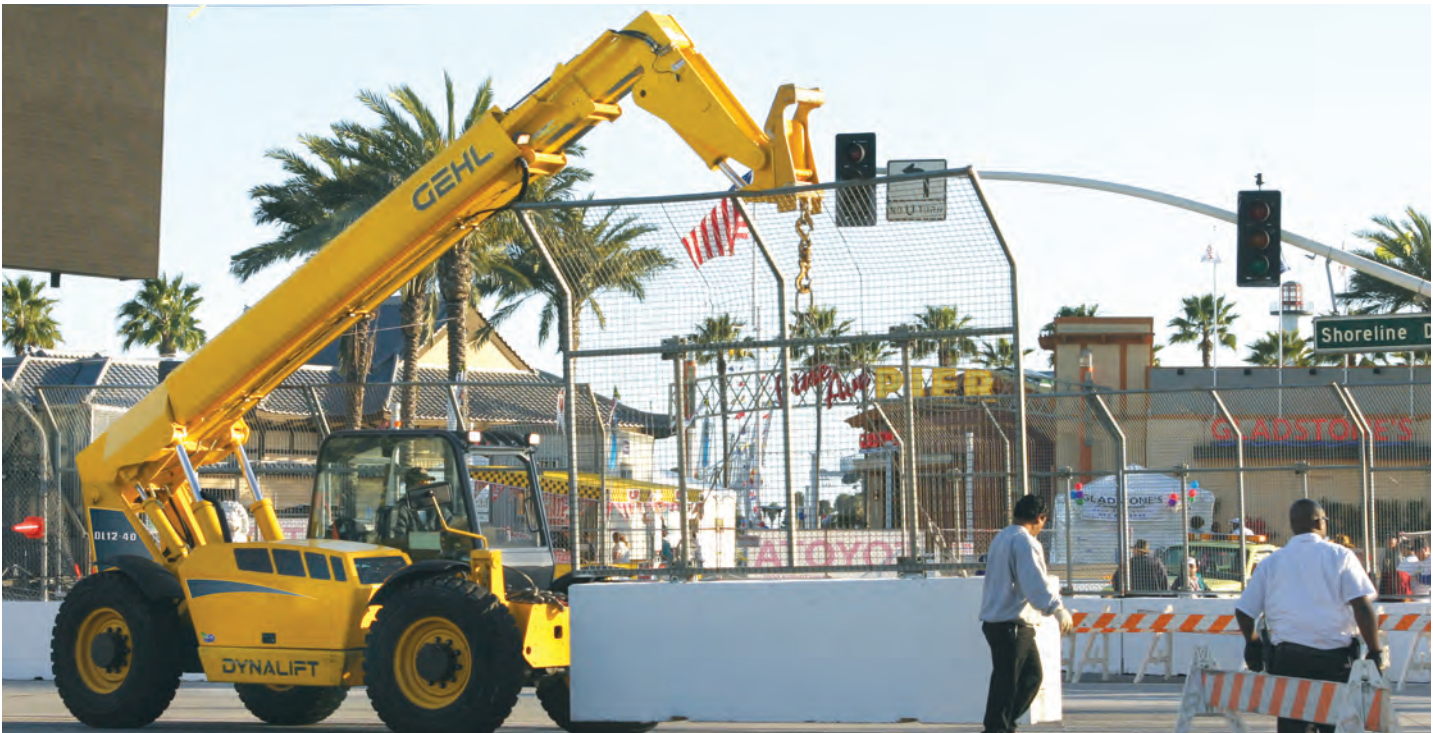
Gehl's telescopic handlers enable the Grand Prix Association of Long Beach to construct the 1.97-mile track for race weekend, which requires 14 million pounds of concrete blocks, four miles of fencing and 17,000 tires bolted together. Gehl is the official construction equipment supplier for the event. (Photograph provided by Gehl)
