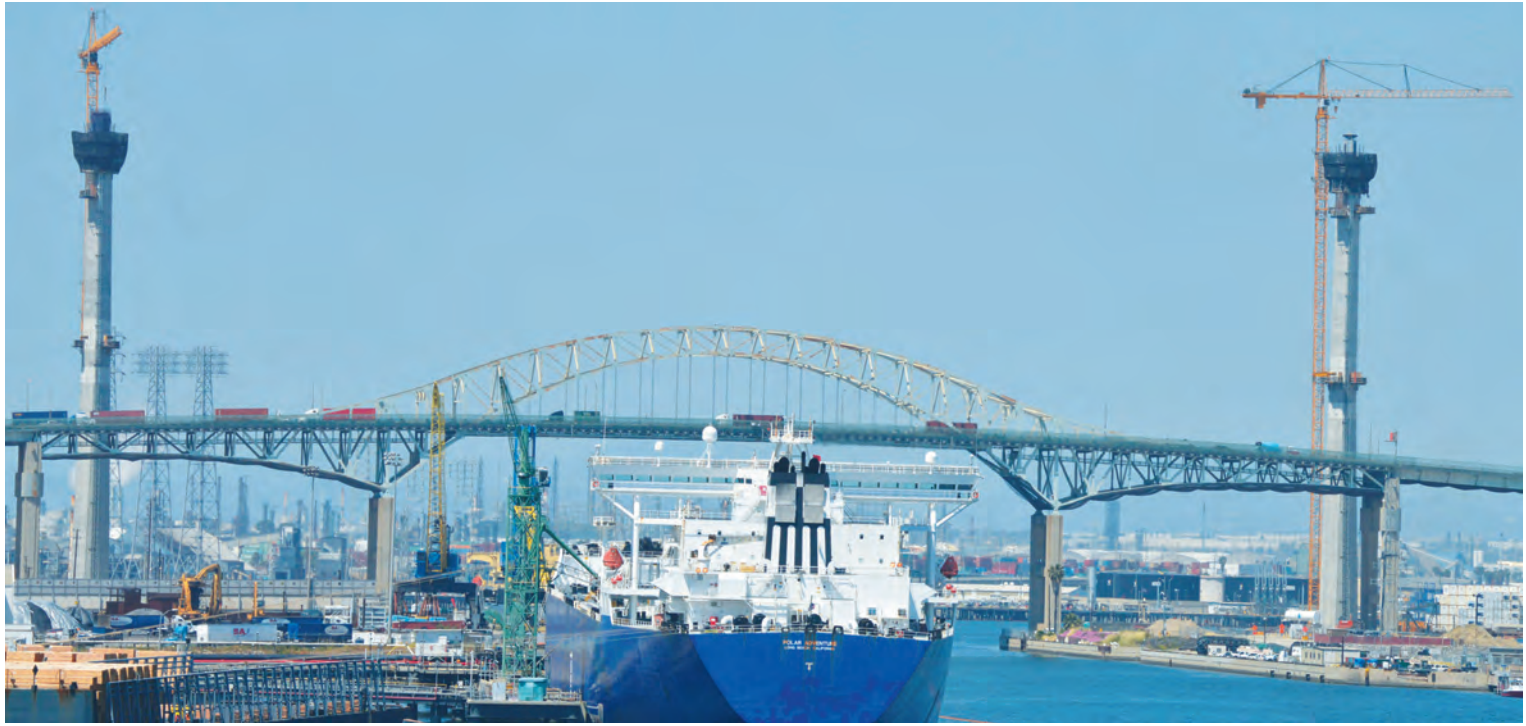
Two towers under construction rise high above the Gerald Desmond Bridge providing a preview of the massive scale of its replacement, which will rise more than 200 feet above the water. (Photograph by the Business Journal’s Larry Duncan)
