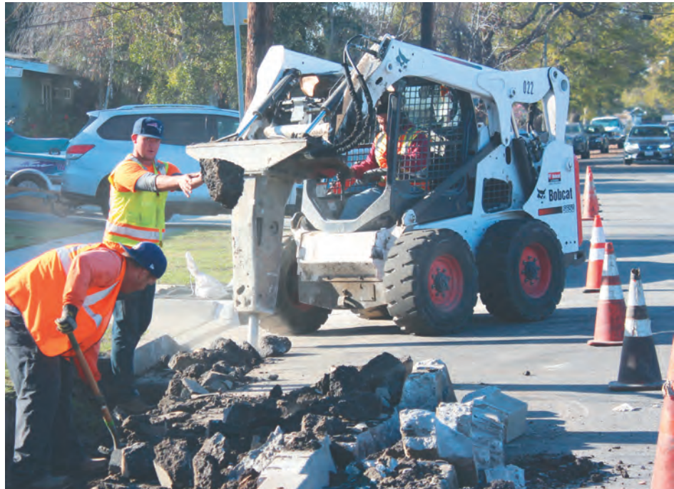
As part of Measure A-funded road work, portions of the gutters and curbs on Stevely Avenue at E. Mantova Street are being replaced. Public Works Director Craig Beck said the first year of Measure A was a success, will all street slurry projects being completed. (Photograph by the Business Journal’s Brandon Richardson)
