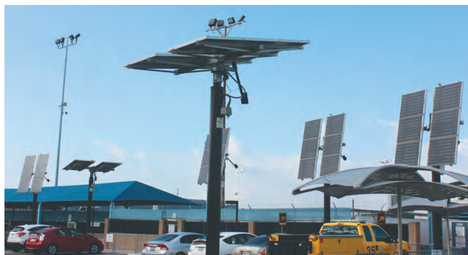
Solar panels at the Long Beach Airport provide plug-in power for electric vehicle charging stations. (Photograph by the Business Journal’s Brandon Richardson)
