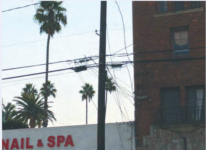
Wires hang from this utility pole located across the street from Gallagher's Pub & Grill on East Broadway. Such wires can pose safety concerns to the neighborhood, including increased risk of fire. High winds are more likely to disconnect poorly maintained wires and down power lines, resulting in damage to private property. (Photograph by the Business Journal's Pierce Nahigyan)
