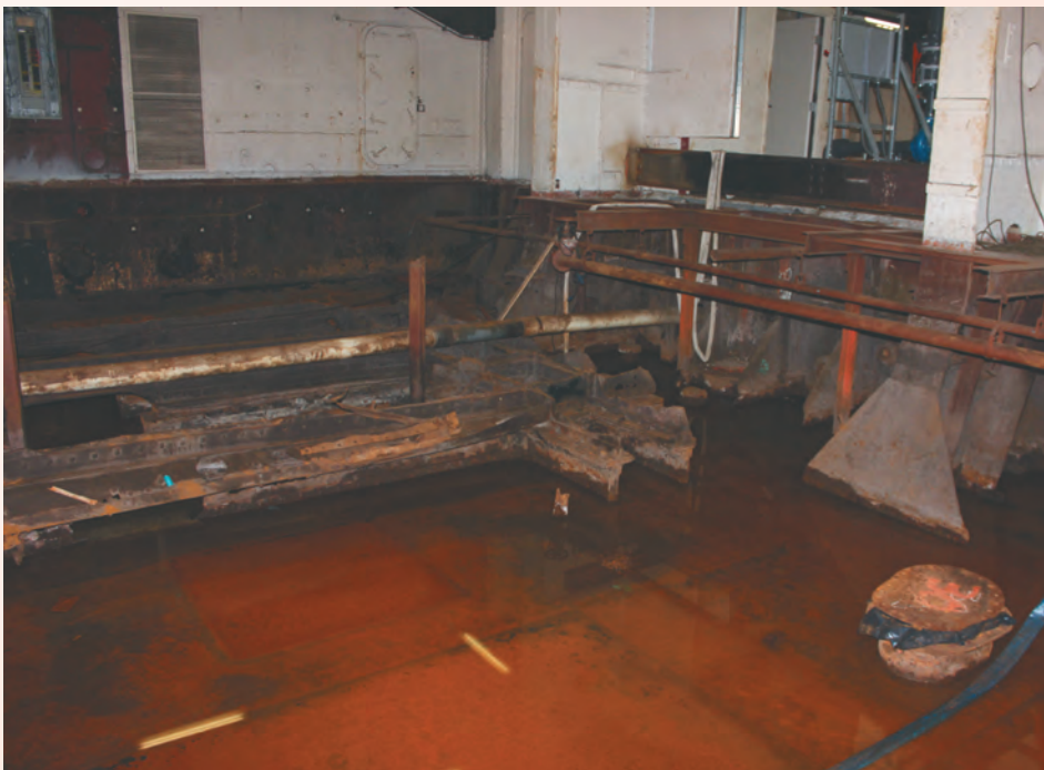
Urban Commons has torn out the flooring and begun patching leaks and treating the corroded steel below the ship’s exhibit hall. When repairs are complete, Chief Development Officer Dan Zaharoni said, the area may be converted into a new kind of space. “We have a lot of ideas about what to do, so this one’s going to take a little bit longer,” he said. “We’re not just going to slap everything back together and start charging for it. I’d rather wait an extra year and create an amazing experience (Photograph by the Business Journal’s Brandon Richardson)
