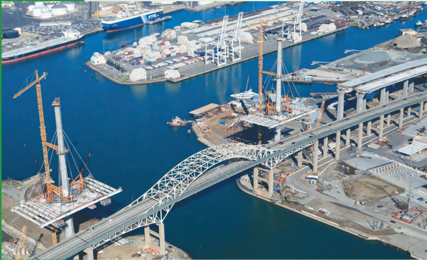
The replacement for the existing Gerald Desmond Bridge is under construction at the Port of Long Beach. At left, the main span of the new bridge rises 205 feet over the harbor, while the Gerald Desmond’s water clearance is 155 feet. The higher structure will allow larger vessels to pass beneath it. (Business Journal photograph by John Robinson)
