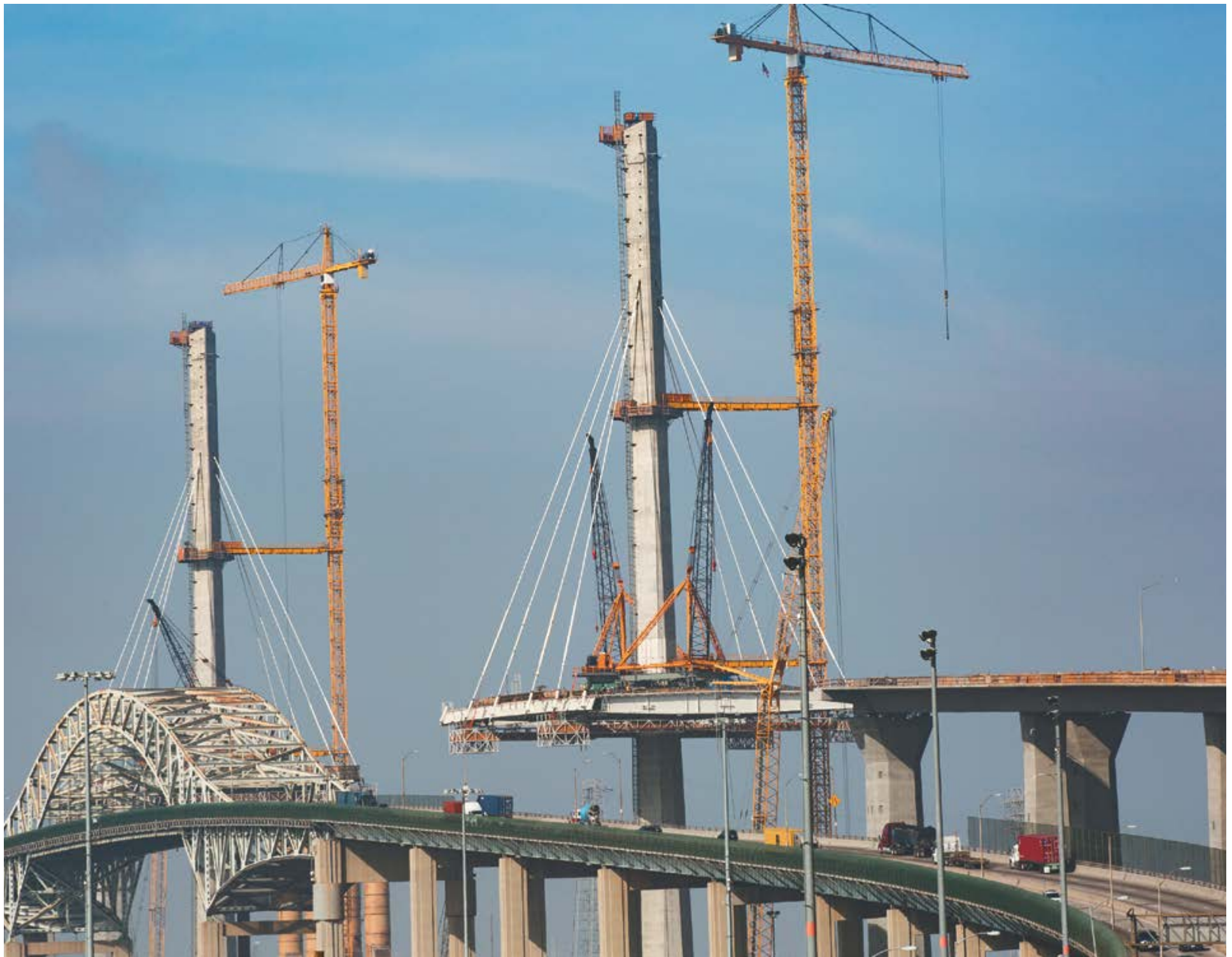
The first cables connecting the towers of a new bridge to its main span have been strung over the entrance to the Port of Long Beach's inner harbor. The structure is replacing the existing Gerald Desmond Bridge, pictured in the foreground, which is reaching the end of its intended lifespan. (Photograph provided by the Port of Long Beach.)
