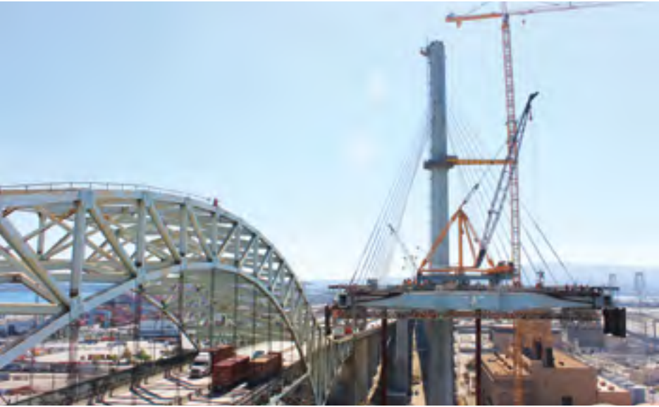
While the Port of Long Beach is moving full steam ahead with the Gerald Desmond Bridge Replacement Project, officials are concurrently developing methods to demolish the old bridge. Duane Kenagy, capital program executive with the port, said there are two options: To demolish the old bridge in the reverse sequence in which it was built, or to lower segments of it onto a barge to be disassembled offsite. (Photograph by Brandon Richardson)
