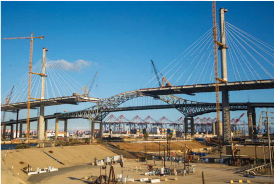
The replacement for the existing Gerald Desmond Bridge, pictured with a bluish-green arch in the background, is expected to be complete in mid-2020. As depicted here, the new bridge is cable-stayed, featuring 515-foot towers and three lanes of traffic in each direction, as well as a path for cyclists and pedestrians. (Photograph courtesy of the Port of Long Beach)
