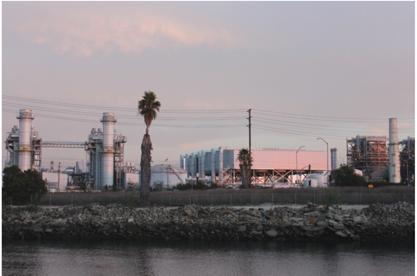
The production of cleaner energy at the AES Alamitos Energy Center in Southeast Long Beach is drawing nearer. The upgraded facility features two gas turbines, which will utilize compressed air and natural gas to create electricity. The facility includes two heat recovery steam generators (two stacks pictured at left), as well as a state-of-the-art air-cooled condenser (rectangular structure at center). The facility's old smoke stacks, such as those pictured at right, are to be demolished. (Photograph by Brandon Richardson)
