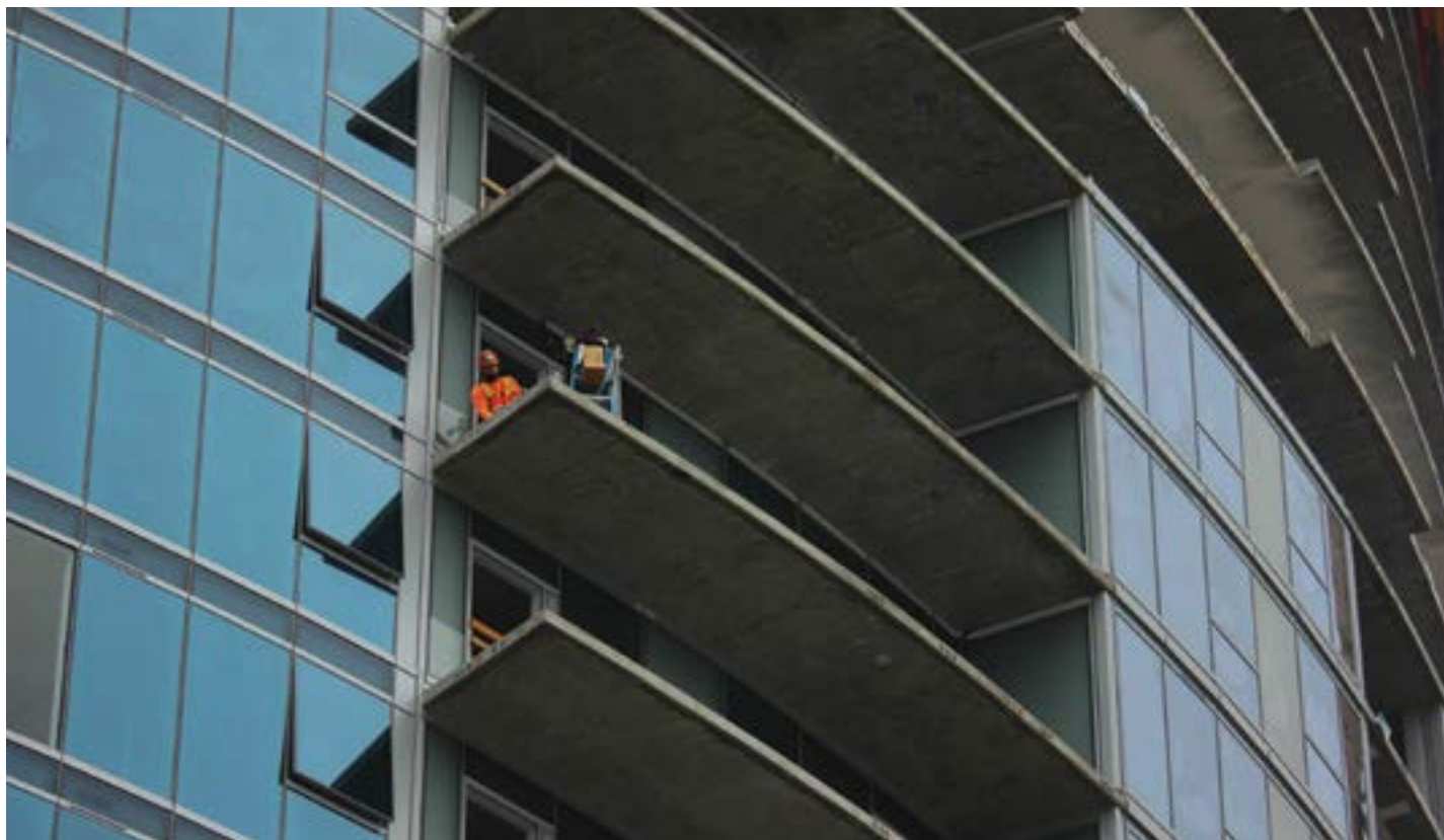
A construction worker seals a crevice on the 14th floor of the Shoreline Gateway development, which will soon be the city's tallest building at 35 stories. Photo by Brandon Richardson.
